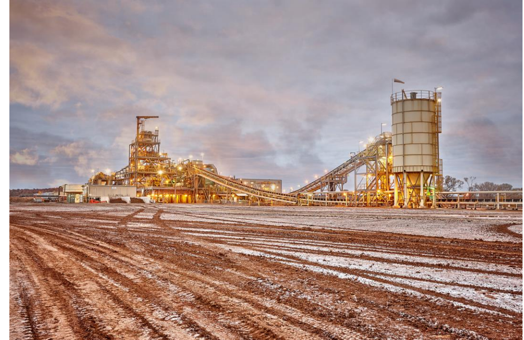
Mt Morgans Processing Plant
