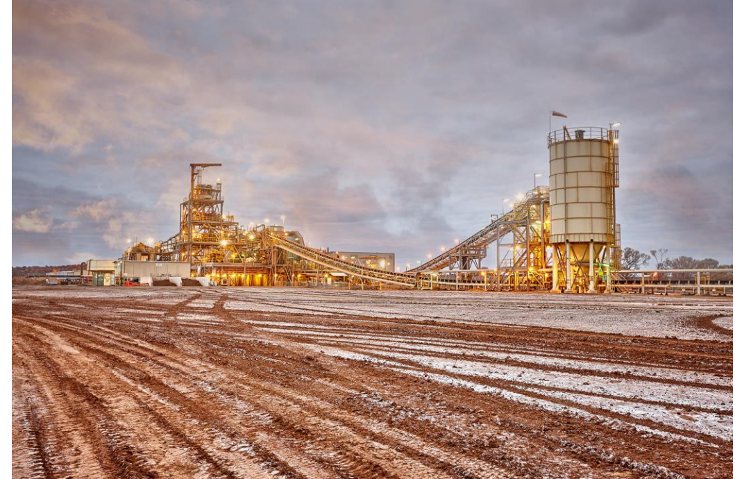
Mt Morgans Processing Plant
