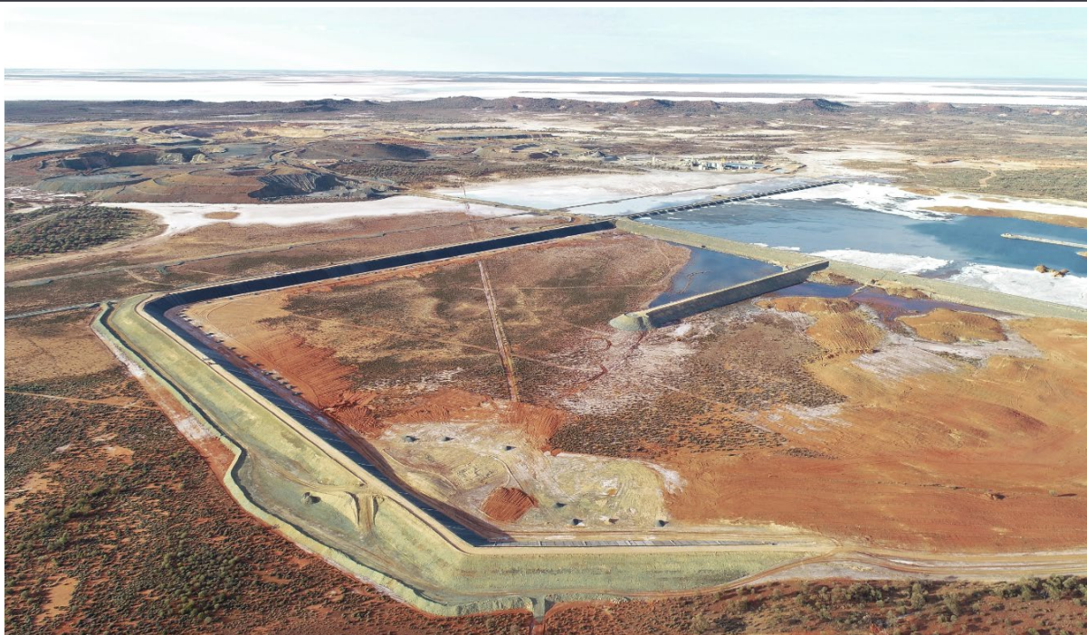
Figure 5: Aerial photograph of the near-complete second cell of the tailings storage facility located adjacent to the treatment plant. The Jupiter open pit is seen in the upper left of the photograph.
